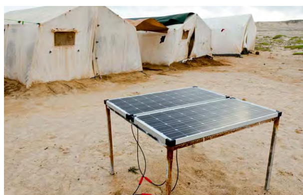
One of the three solar power stations that were purchased for the electricity supply of our field stations; here at Boa Esperança field station.
